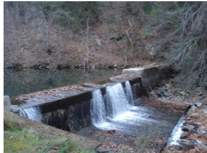
Appalachian Utilities, Inc.
