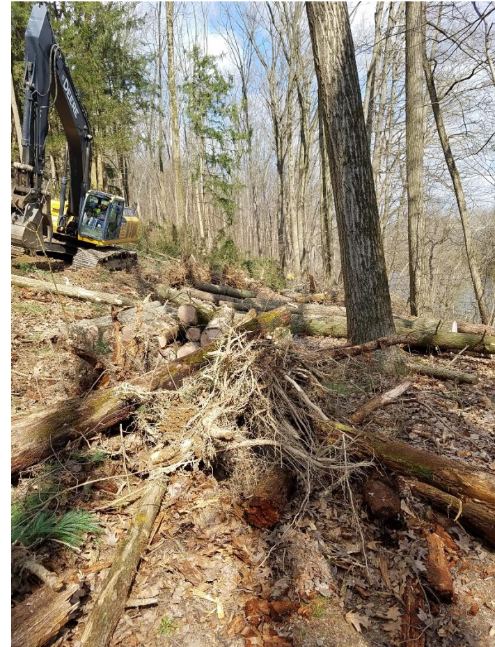
Area to be cleared
