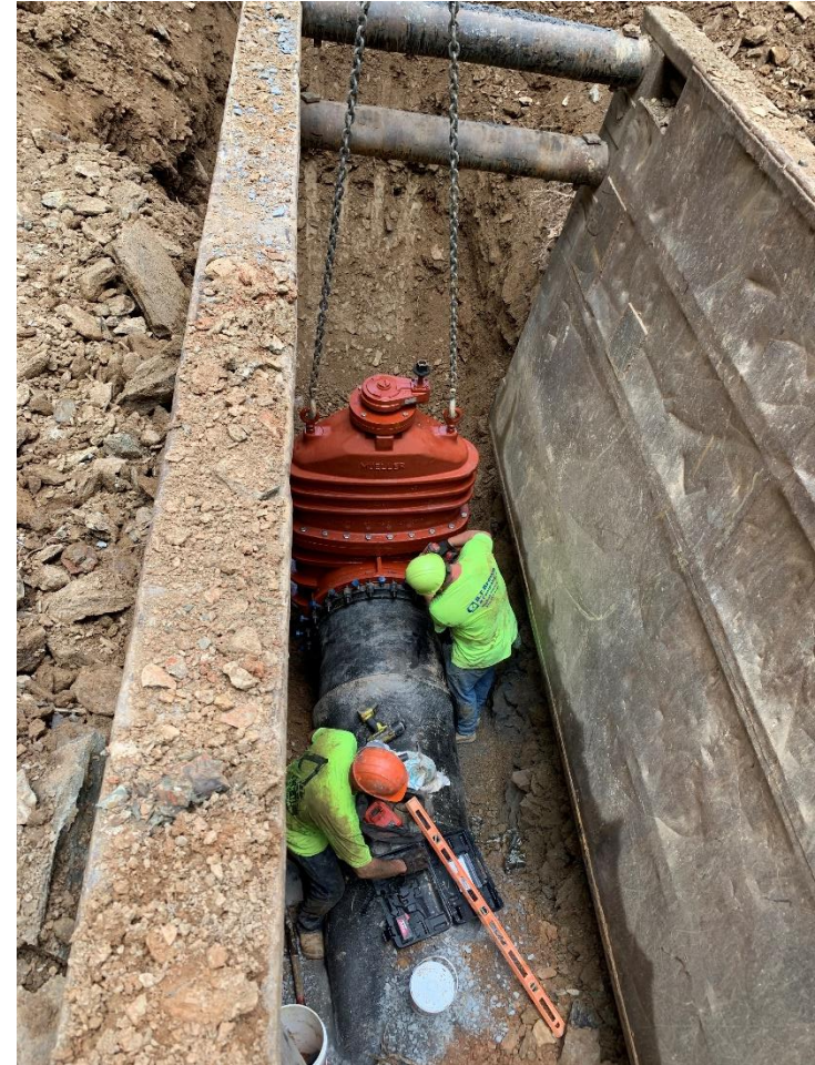
Installation of 30" gate valve
