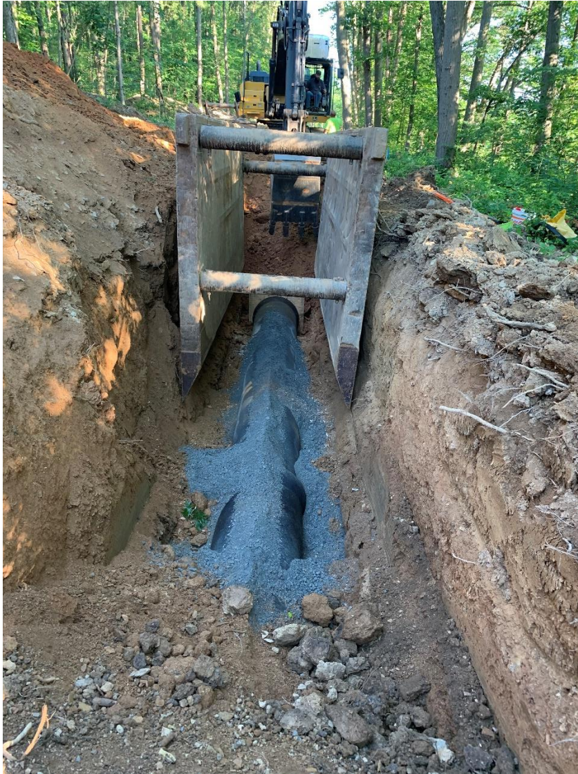
Installing 30-inch pipe
