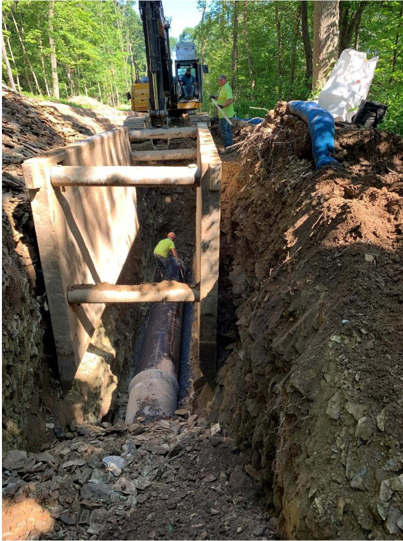
Checking grade level
