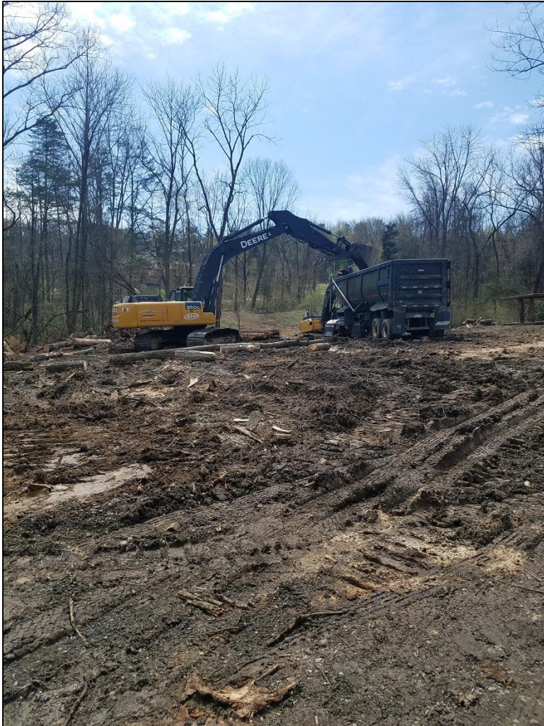
Clearing and grubbing right-of-way
