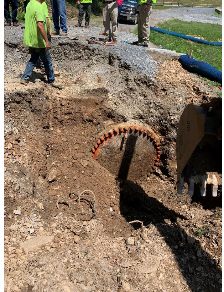
Uncovering the 48" blind flange
